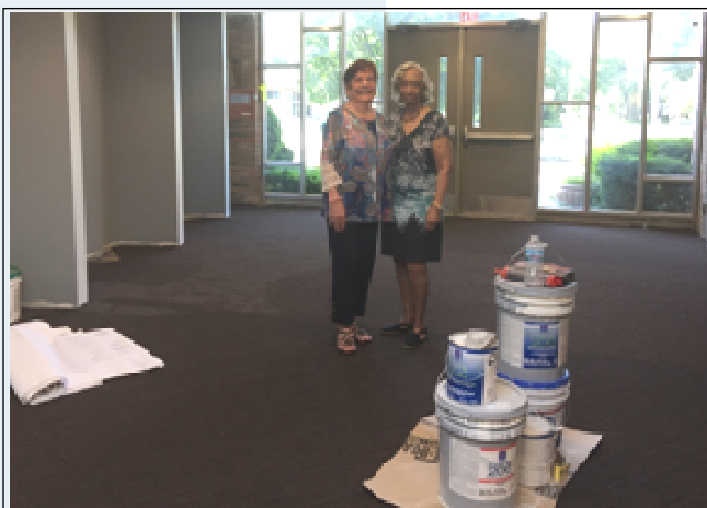
Our vestibule under construction.
